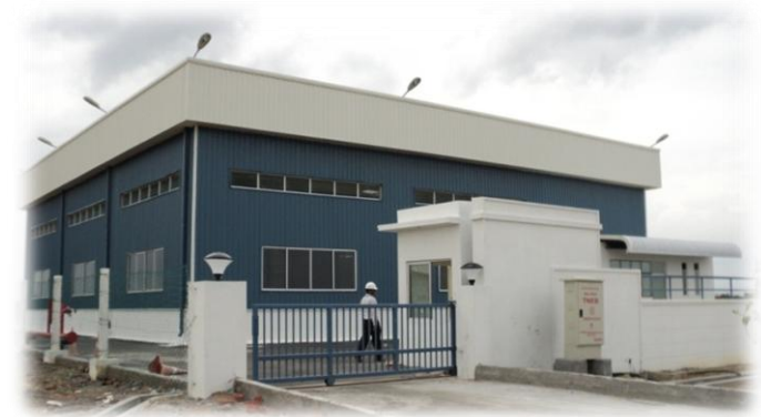
Grundfos Factory Shed
