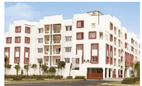
Completed institution buildings and residential block
